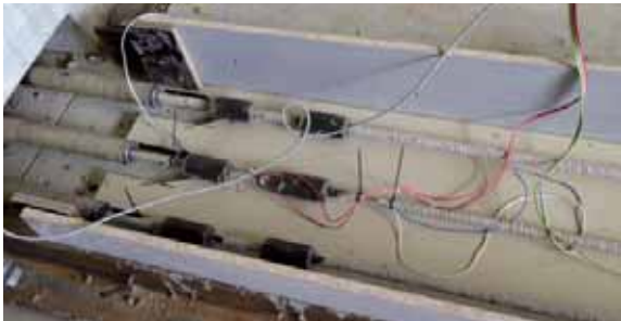
Ceiling panel: preparing reinforcement pre-stressing and measuring equipment
