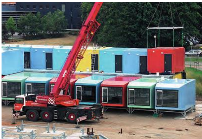
Obr. 85: Proces osadenia objektov Space-box na pozemku. ( Zdroje: SCHITTICH, CH.. Building simply two, s.23.; HOLLAND COMPOSITES. Prefabricated living modules [online]. )
