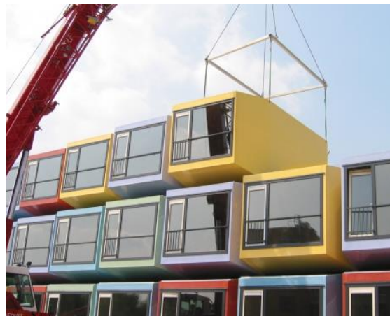
Obr. 85: Proces osadenia objektov Space-box na pozemku. ( Zdroje: SCHITTICH, CH.. Building simply two, s.23.; HOLLAND COMPOSITES. Prefabricated living modules [online]. )
