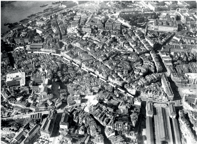
Img. 1. Aerial photograph of Porto 1939-1940 with highlighted Street Mouzinho da Silveira (Source: Foto Beleza )
